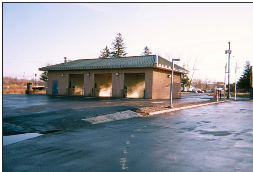
Photograph 6: Rear of car wash building, showing drainage onto street.
